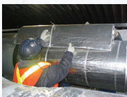
Cryogel Z insulation rolls delivered, cut to size, and installed.
