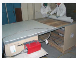
Cryogel Z insulation rolls delivered, cut to size, and installed.
