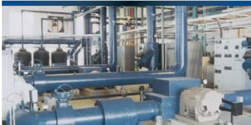
FOAMGLAS® insulation is ideal for low temperature applications—including chill water piping and equipment.
