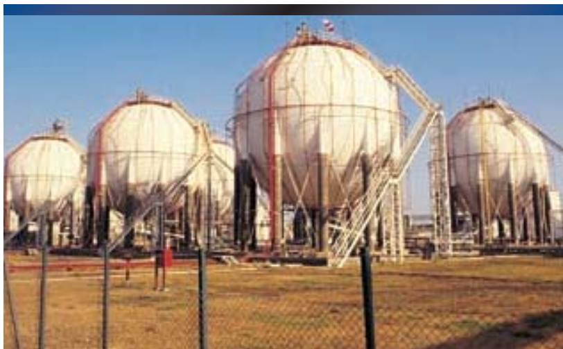
All-glass FOAMGLAS® insulation is commonly used on chemical storage tanks because its high corrosion resistance extends equipment service life.
