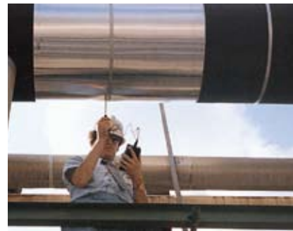
FOAMGLAS® insulation being installed as an "OVERFIT" system.
