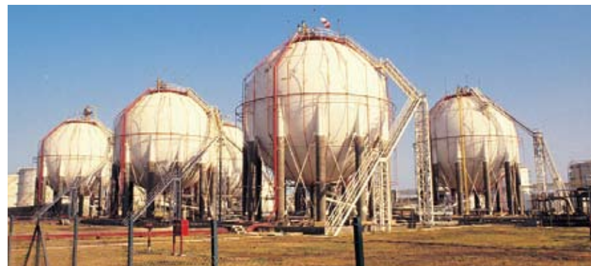
All-glass FOAMGLAS® insulation is commonly used on chemical storage tanks because its high corrosion resistance extends equipment service life.
