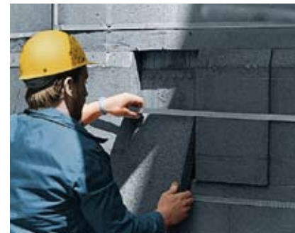
With many FOAMGLAS® insulation projects, an insulation sample is removed after many years of service for testing and replaced with new FOAMGLAS® insulation.
