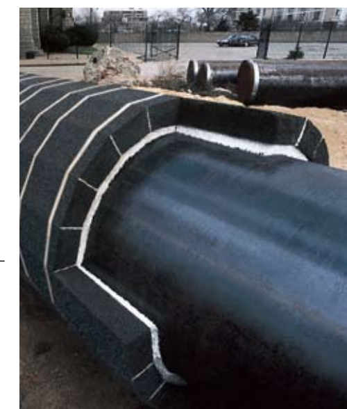
FOAMGLAS® insulation was installed as part of a composite insulation system. It incorporates a one-inch layer of fibrous glass felt material directly around the pipe, covered with FOAMGLAS® insulation.
