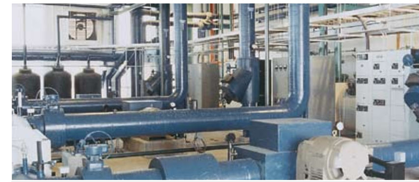
FOAMGLAS® insulation is ideal for low temperature applications—including chill water piping and equipment.
