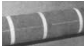
1 FOAMGLAS® Insulation installed with chalk line at three o'clock position.
