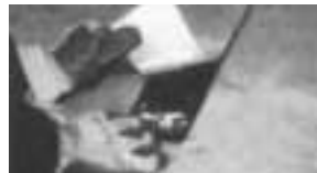
7 Remove release paper from PITTWRAP® jacketing butt strip.
