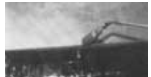
8 Burn off polyester film for distance of 2" on each side of PITTWRAP® jacketing.
