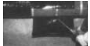
6 Heat remaining half of PITTWRAP® jacketing, pull jacketing around, and make lap seal.
