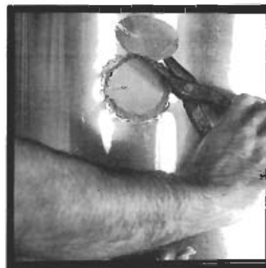
WITH TIN SNIPS CUT OUT COMPLETE HOLE OR DRILL WITH A 2 9/16" HOLE SAW.
