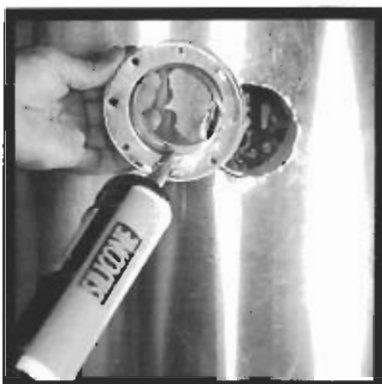
FILL BACKSIDE OF FLANGE WITH SILICONE
