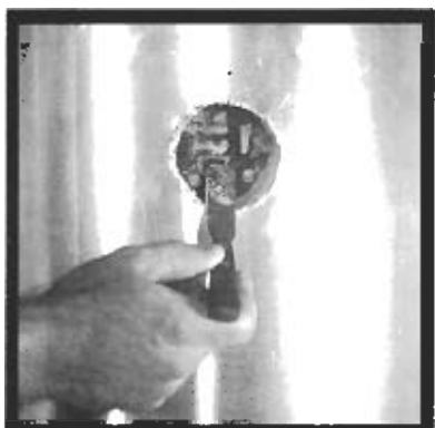
CLEAN OUT INSULATION AS REQUIRED.
