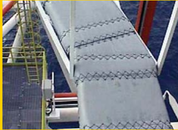
DARMATT J120 Jet fire rated flexible passive fire protection systems
