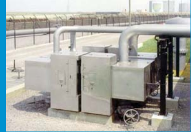
DARSHIELD Rigid and compact passive fire protection enclosures
