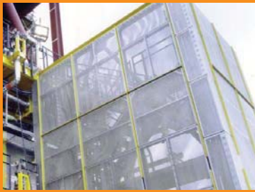
RADIANT HEATSHIELDS DARMET Radiant Heatshield System
