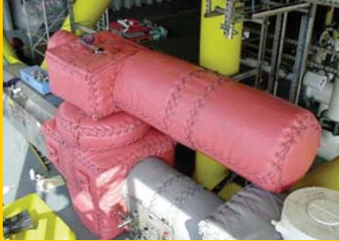
DARMATT Flexible passive fire protection systems
